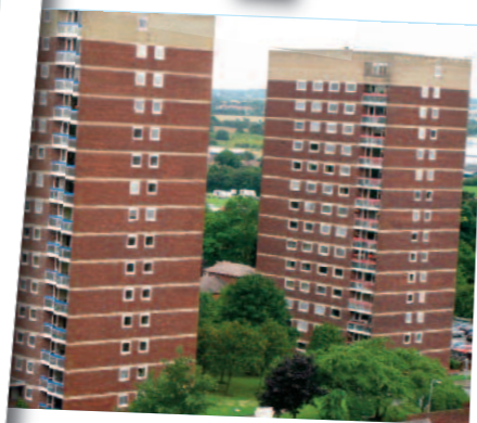
December 2013 - Lift Refurbishment Consultation
